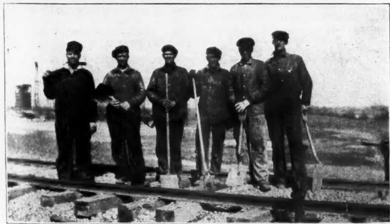
Above, the Bucket; Center, the Screens; Below, the Crew.
